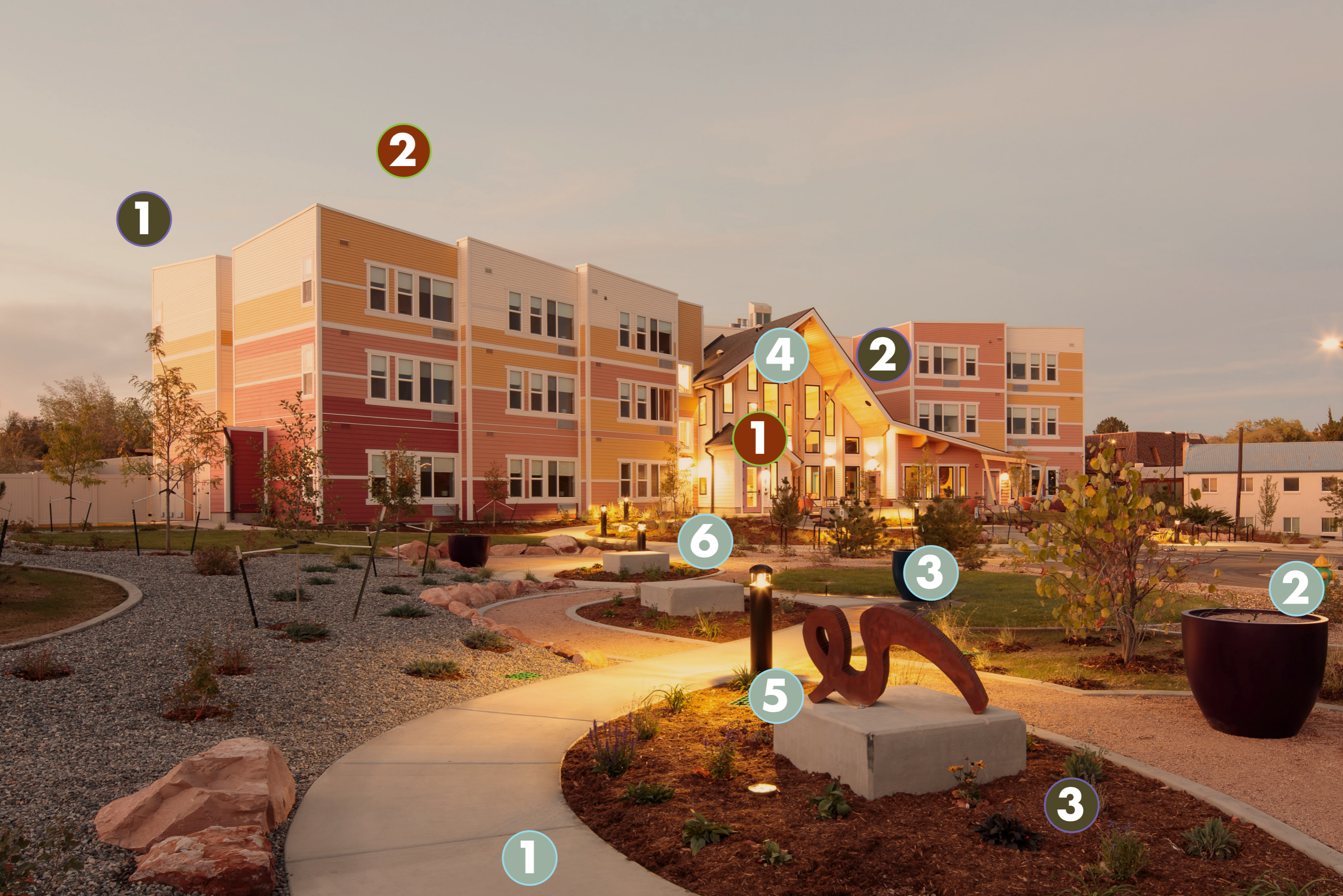
Building exterior and sculpture garden with walking path. Laurel House. Grand Junction, CO. 2020. A supportive housing development for youth exiting homelessness.
